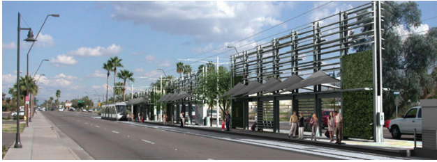
Future light rail station in Phoenix, Arizona
