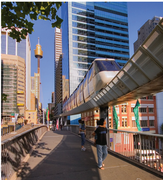
Monorails and their stations are completely aerial.
