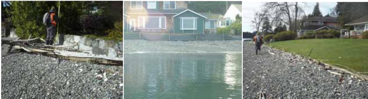
**Figure 4-40: Overtopped bulkheads from RP1 wake wash at 12.75 ft MLLW water level. From left to right: 3698, 3780 and 3804 at Point White Dr.**
