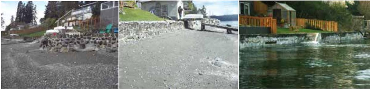
**Figure 4-41: Overtopped bulkheads from RP1 wake wash at 13.25 ft MLLW water level. From left to right: 3192, 3204 and 3284 at Point White Dr.**
