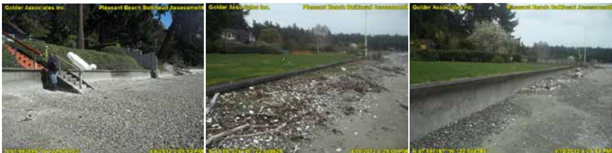
**Figure 4-44: Examples of overtopped bulkheads from SE and SW wind waves. From left to right: 3385, 3861 and 3863 located at Pt. White Dr.**
