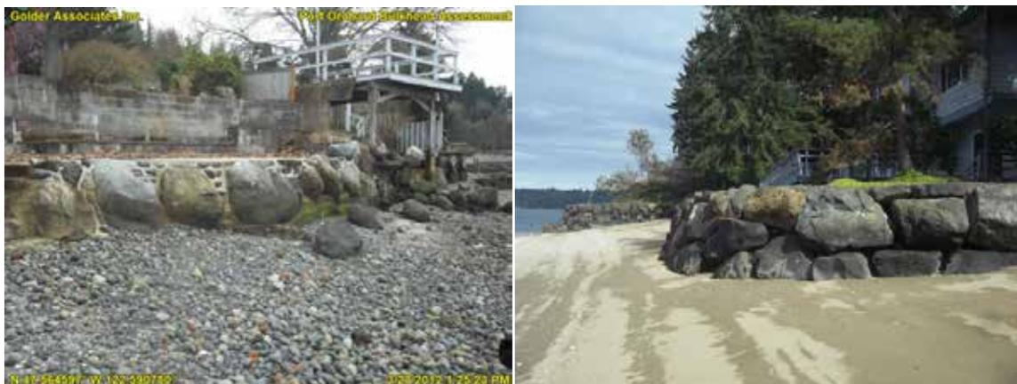
**Figure 4-42: Overtopped bulkheads from RP1 at 12.75 ft MLLW water level. From left to right: 3262 and 6601 Beach Dr E.**
